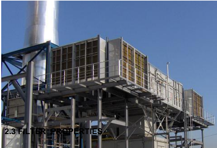
Picture.3- Sample Application of a Combustion Turbine Inlet Air Cooling Unit
