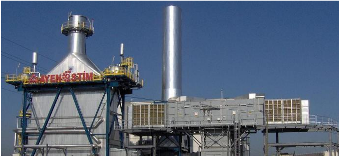
Picture .1- Sample Application of a Combustion Turbine Inlet Air Cooling Unit
