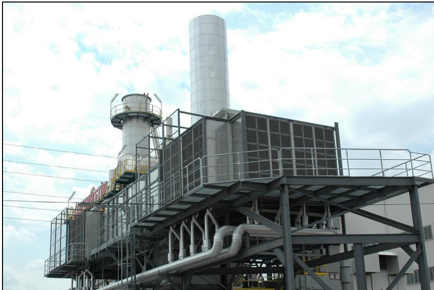
Picture.2- Sample Application of a Combustion Turbine Inlet Air Cooling Unit
